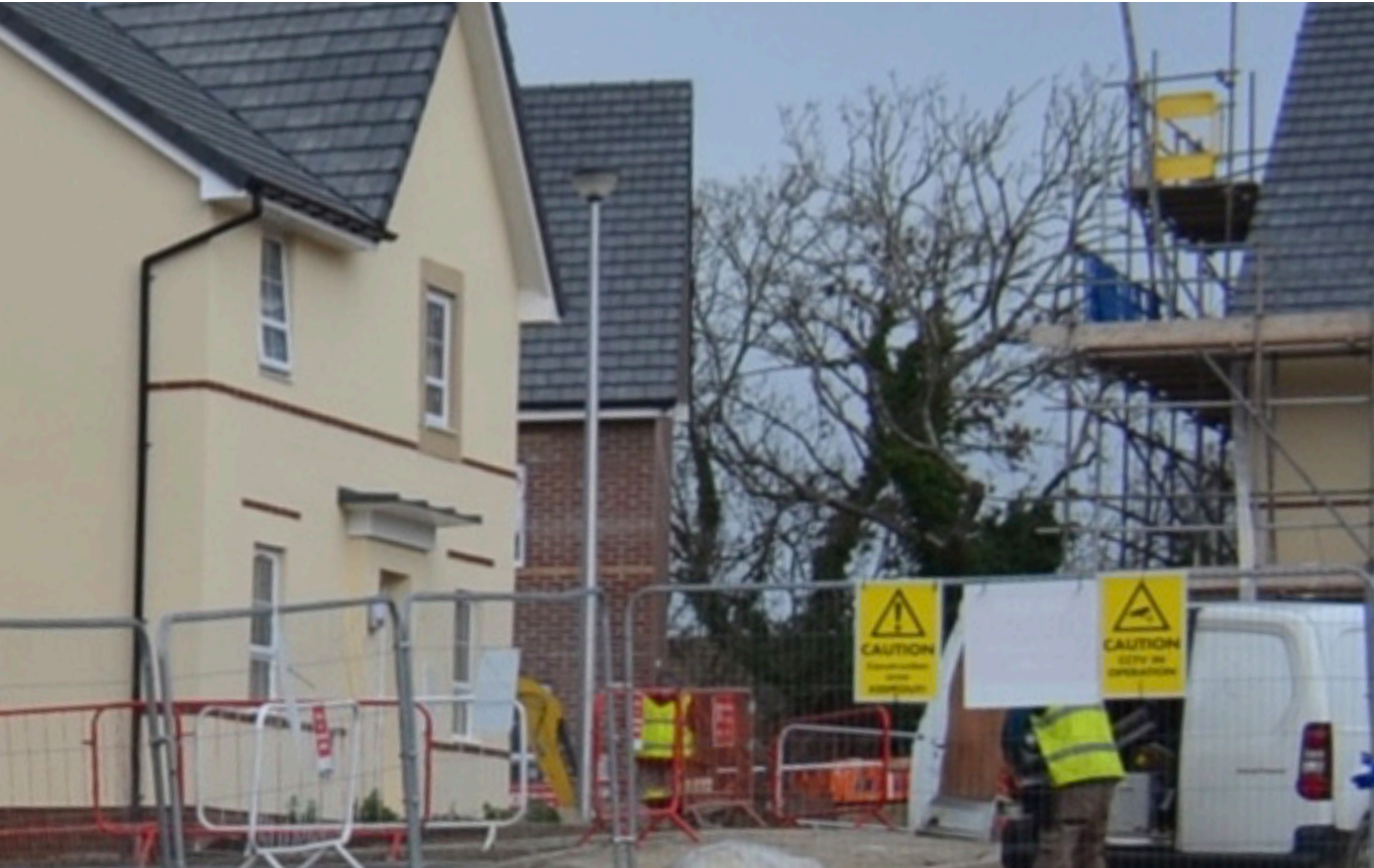
Figure 8: New house building
